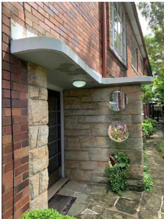
Figure 5 and 6: Main entry door with a curve concrete slab awning over an ashlar sandstone blade wall and curved 'streamlined' plasterwork.
